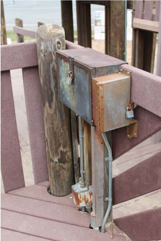
#18 Live electric box within play equipment area.
