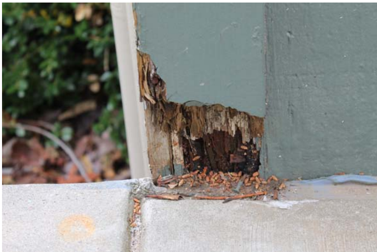
# 57 Rot at foundation.
