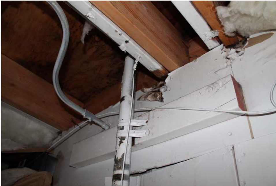
#62 Mold repairs were not done correctly.
