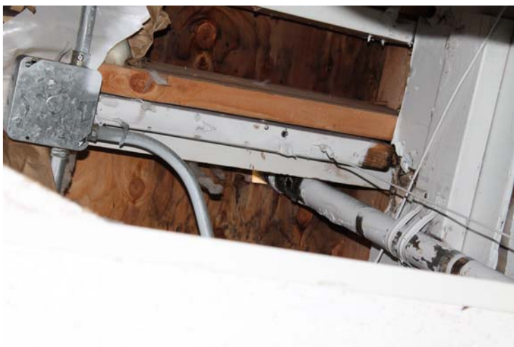
#61 Mold repairs were not done correctly.
