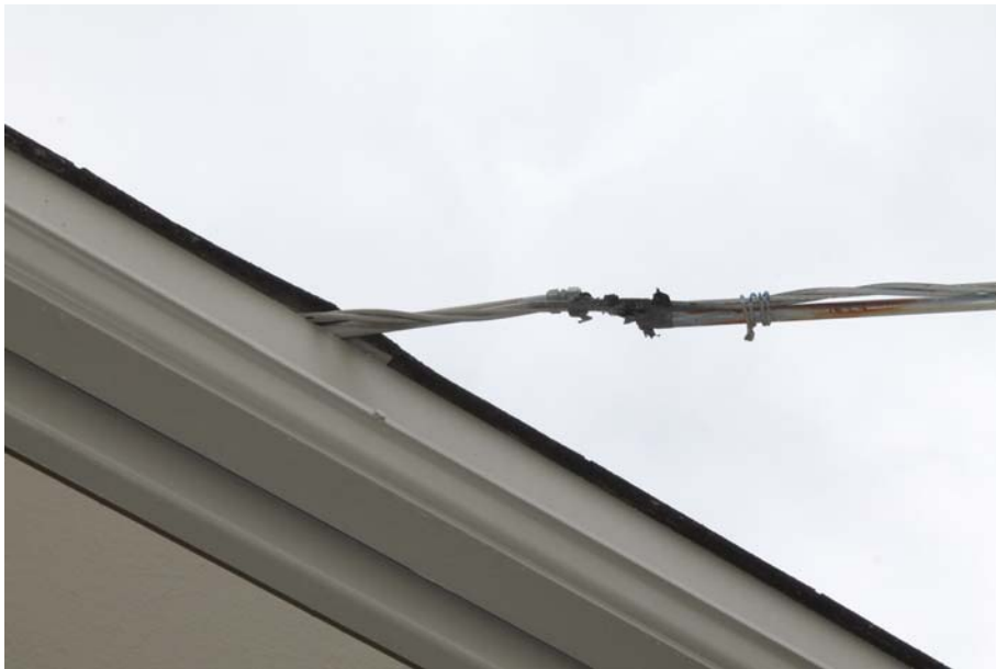
#86 Frayed and broken insulation used to carry 110 volts of electric power. This exposes the live wires to elements. Note also the routing is under the roofing material, no anchors to keep the wires from pulling away.
