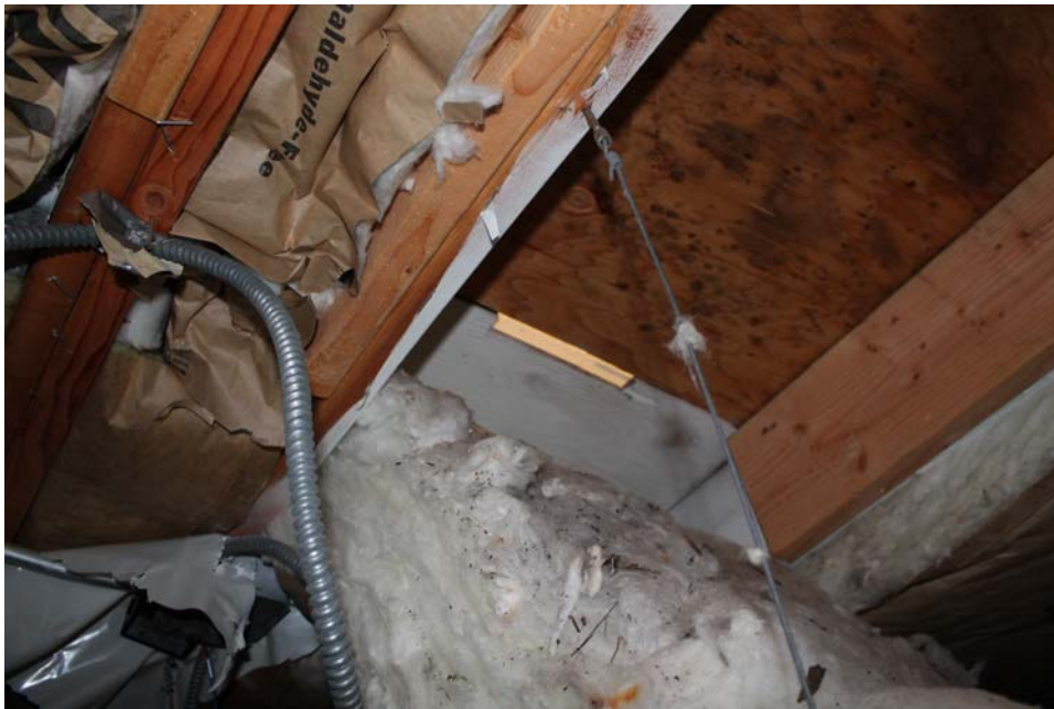
#63 Mold repairs were not done correctly.
