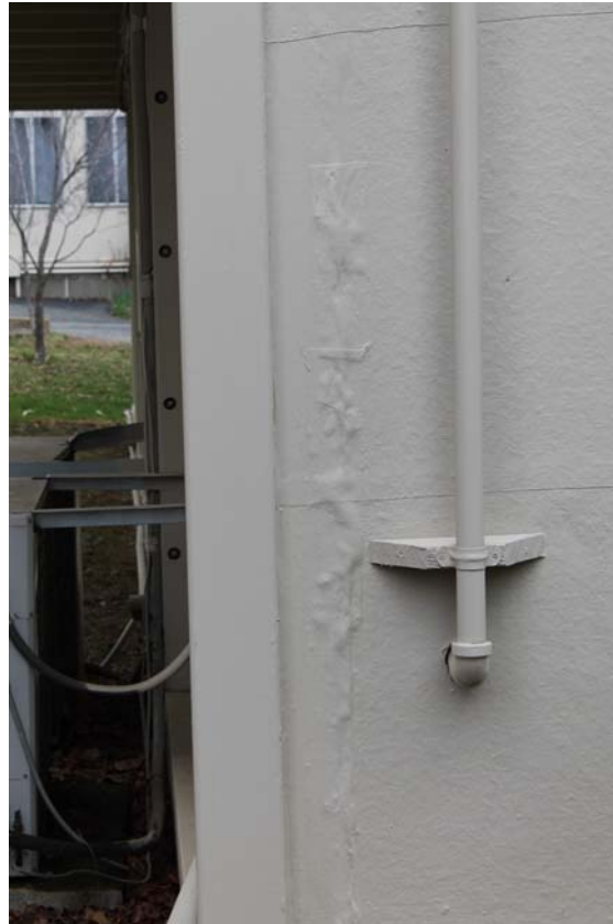
#85 - Siding is separating from wall structure. This is evidence of water penetration to interior of wall structure.
