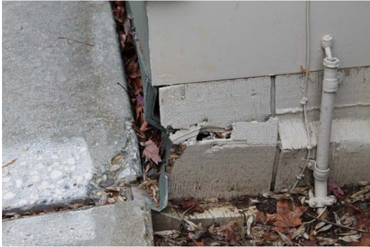
#51 - Siding is separating from wall structure. This is evidence of water penetration to interior of wall structure.
