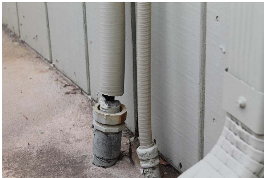
#41 Broken electric conduit at ground level is at risk for high flooding from the adjacent Veteran's Hall parking lot.
