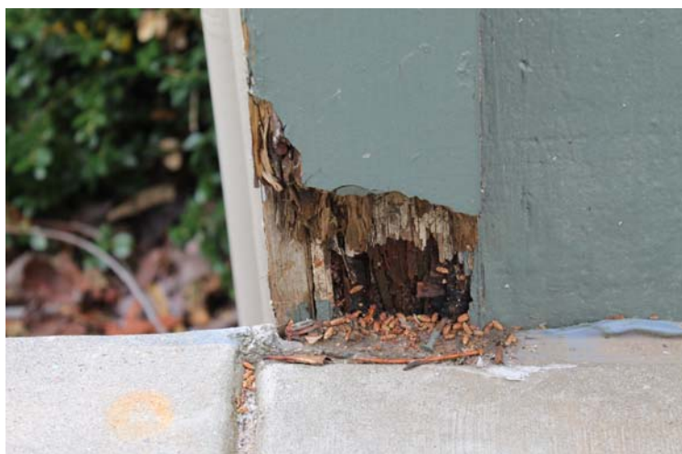
# 57 Rot at foundation.
