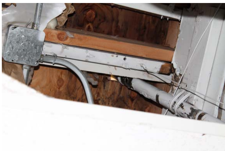
#61 Mold repairs were not done correctly.
