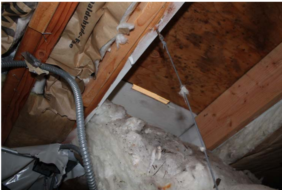
#63 Mold repairs were not done correctly.
