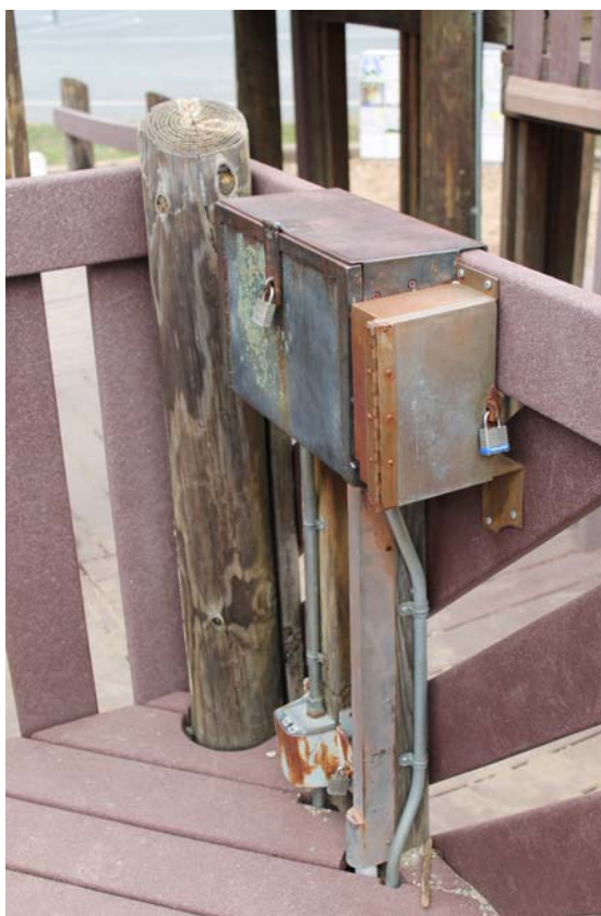
#18 Live electric box within play equipment area.
