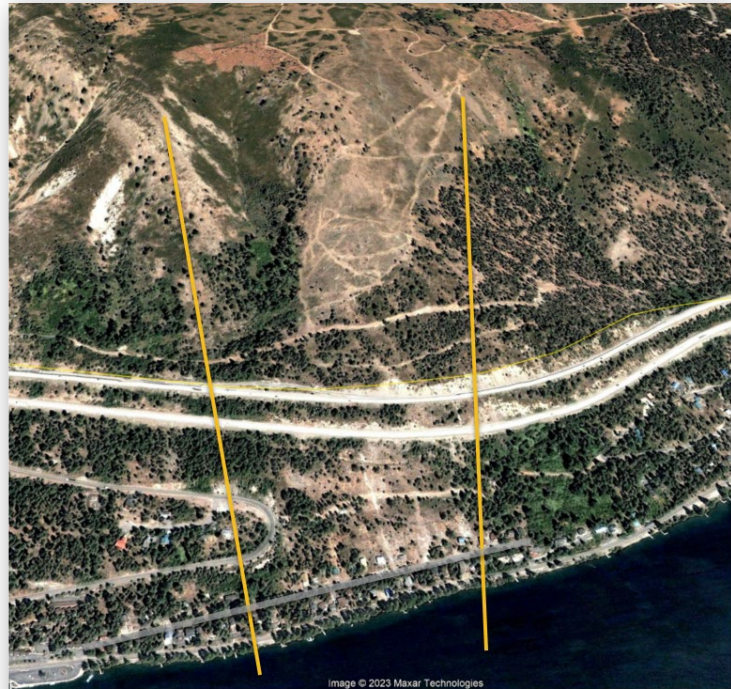
The location specific to this report, 1,500 feet of steep hillside assessed to be at the highest level of risk for erosion and landslides, a location that carries polluted runoff from I-80.
