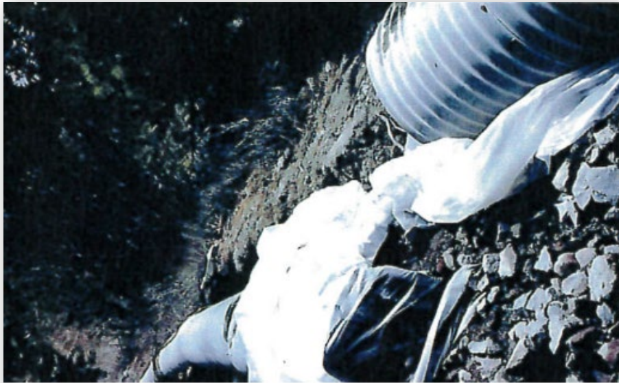
I-80 Drainage Culvert
