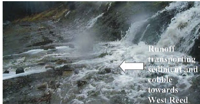
Water and electric utilities buried under unpaved road without drainage mitigation on hillside below I-80, above Reed Avenue West, Donner Pass Road, and Donner Lake.
