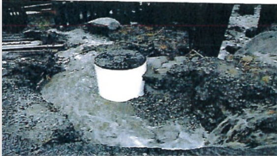
Utility infrastructure on Reed Avenue West
